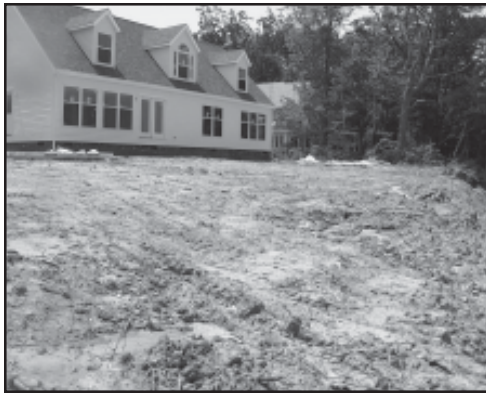
The project in these photos would be considered in violation for excessive land disturbance and clearing of vegetation.
