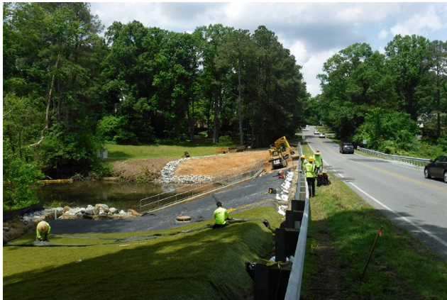
Installation of improvements to Canterbury Dam Source: Timmons Group
